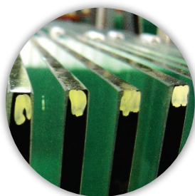
marking after Heat-Soak-Test
